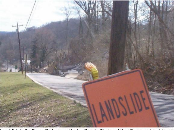
Landslide in the Devou Park area in Kenton County. The toe of the hill was undercut to put in a driveway, and with excess drainage the slope failed. Note the angle of the trees. These sand, silt, clay, and gravel deposits were laid here by glaciers over 125,000 years ago. Photo by Richard Smath, Kentucky Geological Survey.
